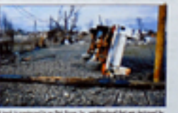
A view of a destroyed home in a New Orleans neighborhood hit by Hurricane Rita.
